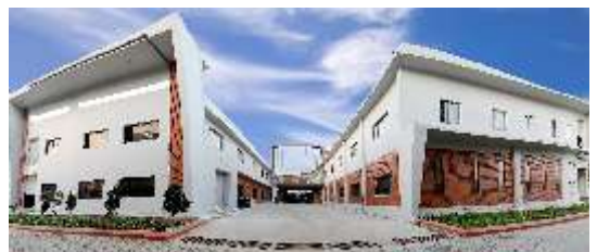
Tempsens Instruments U# II Cable Plant
